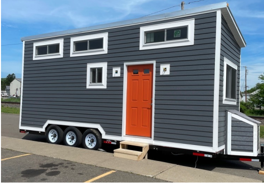
Tiny House built by Owego's Building Trades students
