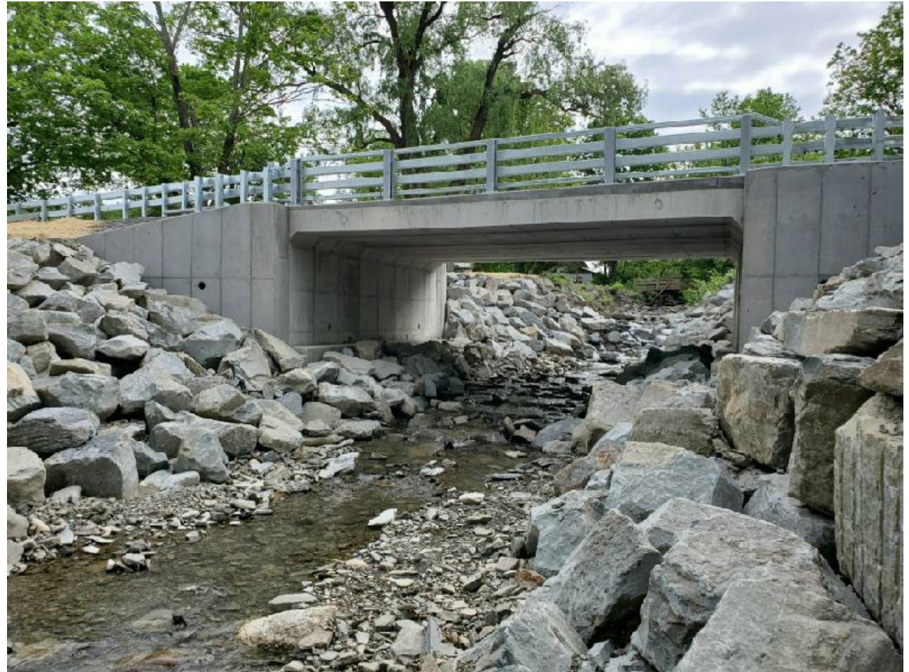
(Gaylord Stream Crossing Replacement project. Owego, NY)
