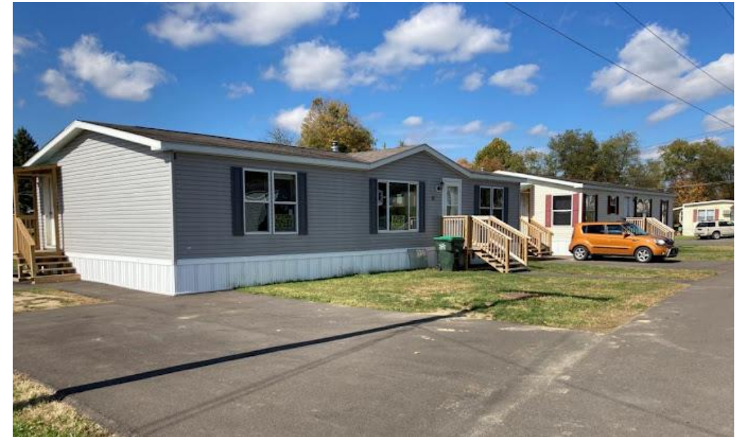
Owego Heights Mobile Home Park
