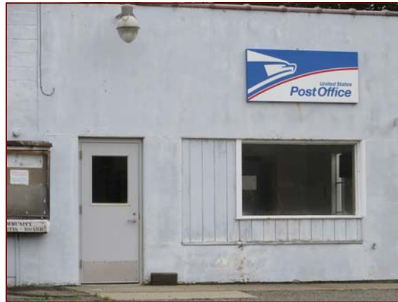
Former Tioga Center Post Office
