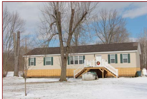
Example of elevated home in the Town of Tioga
